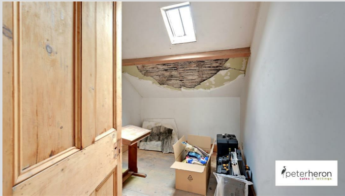
A sloping ceiling with a skylight window.
