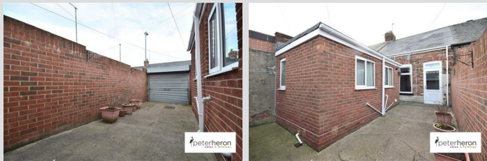
Courtyard to the rear with a remote control roller shutter access door.
