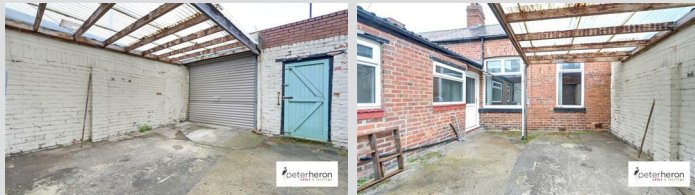
Small area to front and enclosed rear yard with roller shutter access door to carport.
