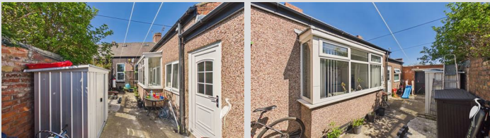
Courtyard with double gates to rear.
