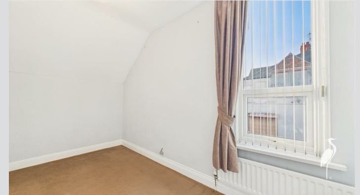
Double glazed window to side and radiator.
