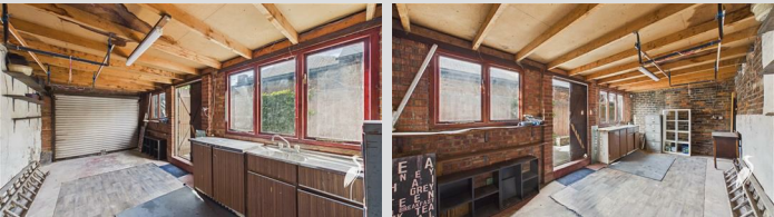
Base units incorporating a single bowl stainless steel sink and drainer. Accessed via roller shutter door. Single glazed windows and door to rear garden.
